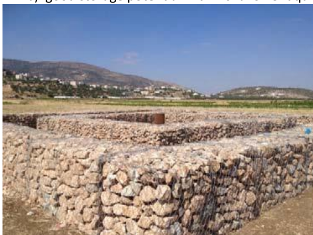
Filtration System - Gabions, around an artificial recharge well
